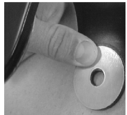
Installing the Stainless Steel Washers
